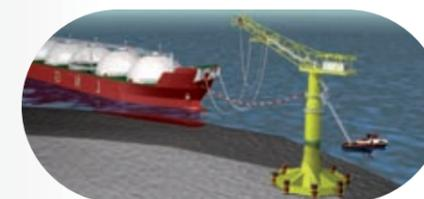
For the more demanding environments, the weathervaning SPM type terminal has been successfully implemented and accepted over the past three decades by the oil and petrochemical industry.
