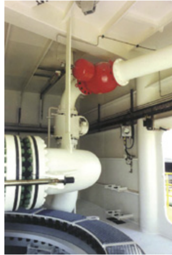
The surge relief valves are protected inside the deckhouse together with the swivel and as shown in this picture, together with the flexible joints and the main bearing.
