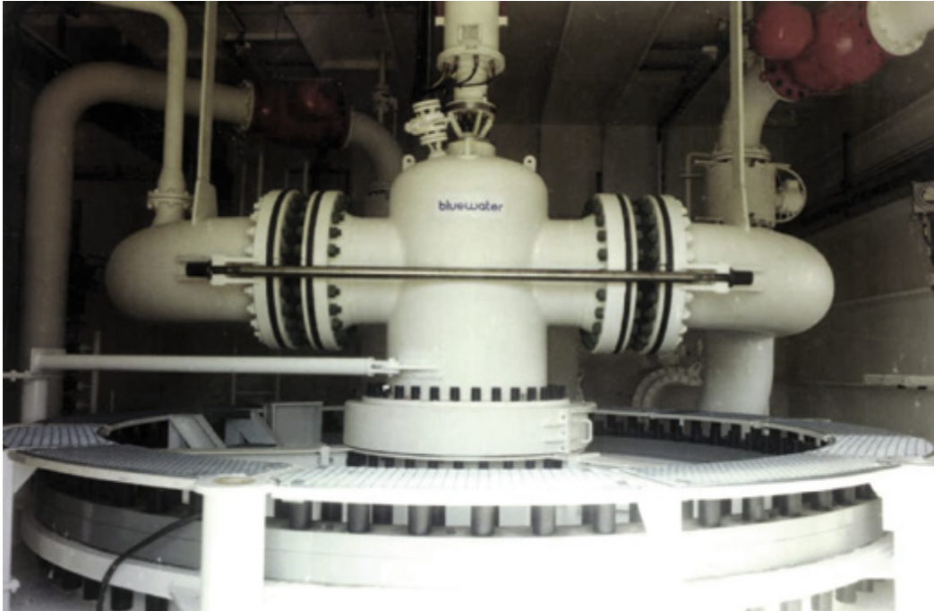
Ocenca, Colombia, TLU-2 Terminal, Interior deckhouse with Bluewater swivel
