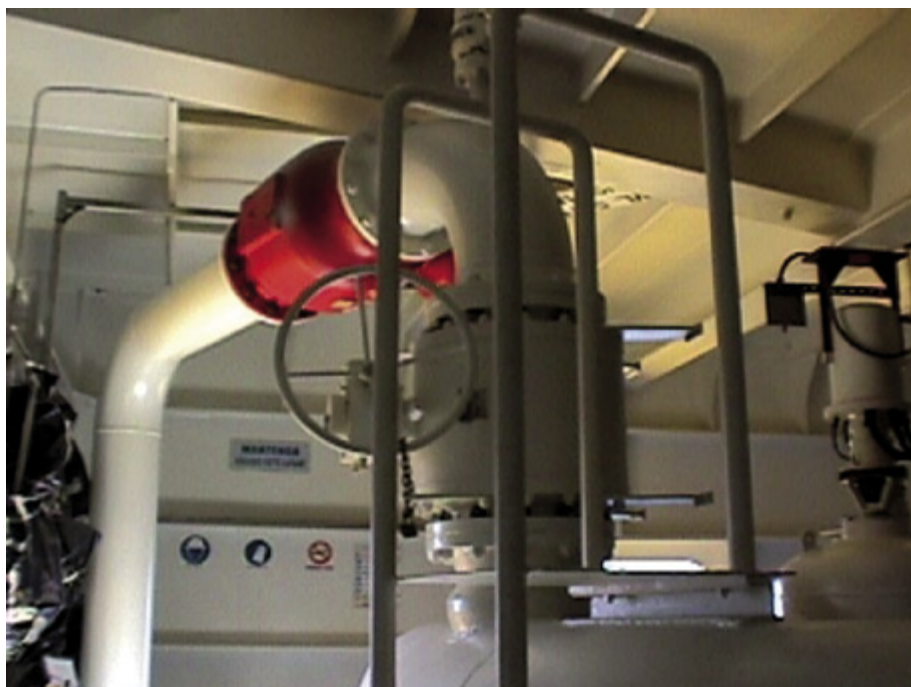
Ocensa, Colombia, TLU-2 Terminal; Piping for Surge Relief System inside deckhouse
