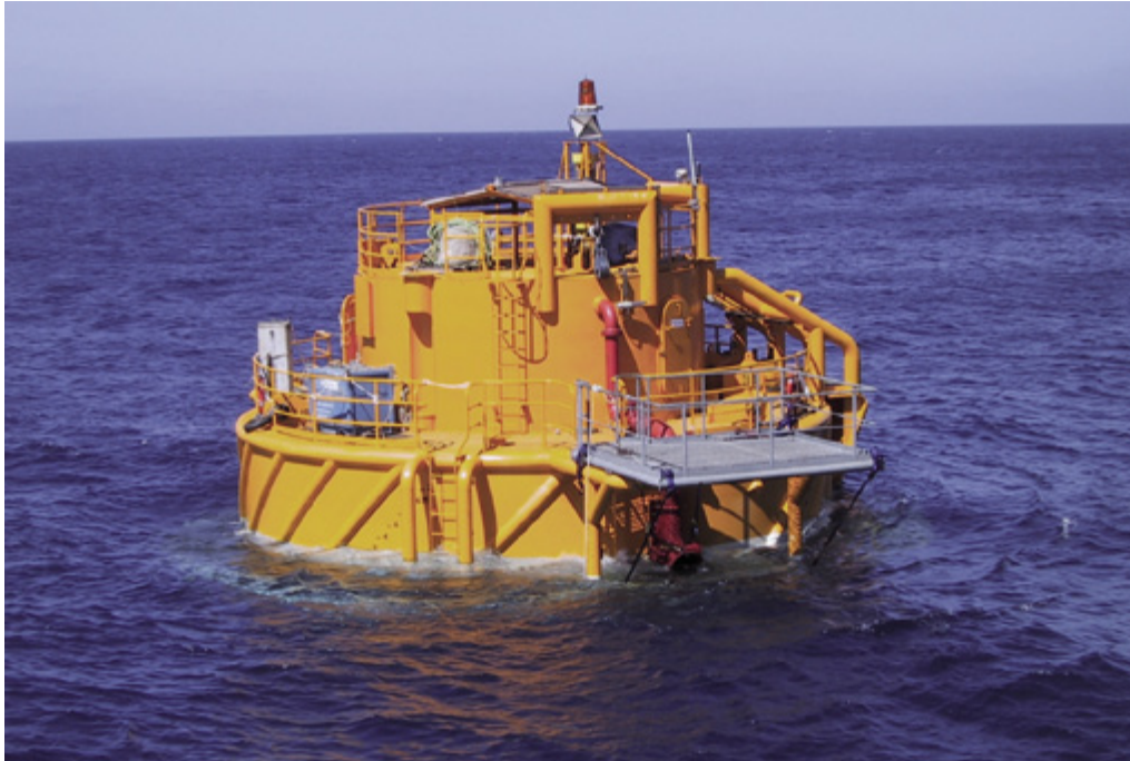
Apache Stag Field, Australia, Turret Buoy during installation
