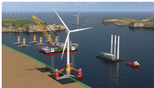
Assembly with Bluewater's TIF (Transport and Installation Frame)
